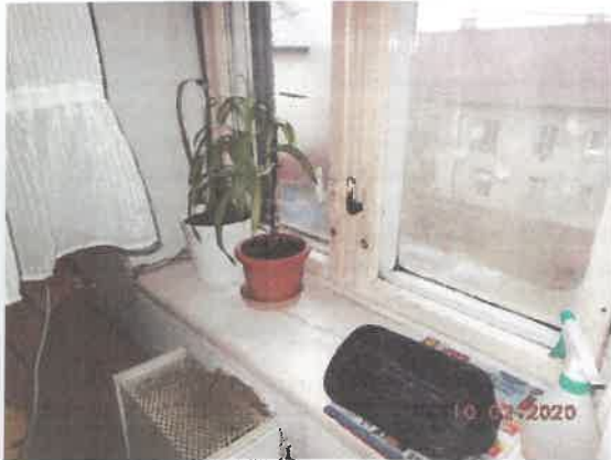
Detail okna v kuchyni
