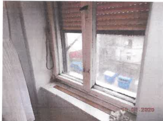
Detail okna v kuchyni
