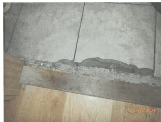
Detail podlahy kotolne 1.05
