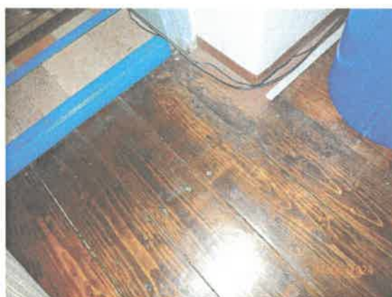
Detail podlahy kuchyne – palubovka
