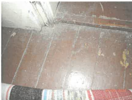
Detail podlahy kuchyne - palubovka
